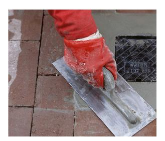
A non-shrink concrete designed for the surface reinstatement of 'picture frames' or fillets around access covers and surface areas around street furniture.
